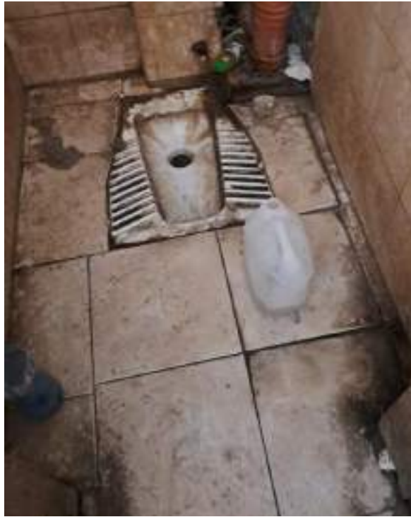
A toilet at the facility. At night, the men are forced to urinate out the window.
